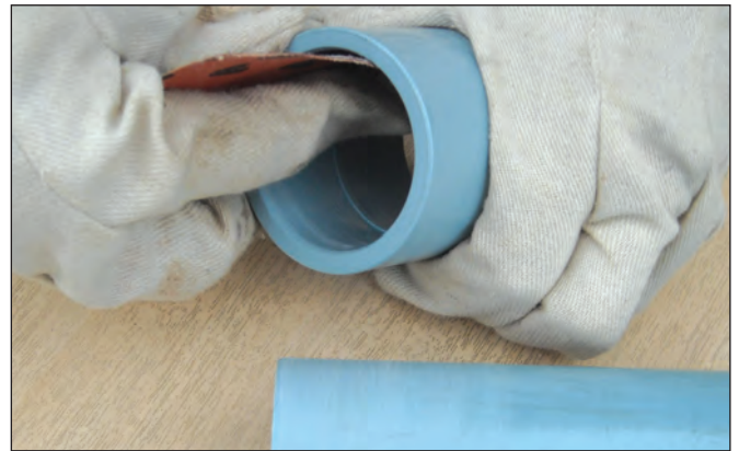
4. Abrade pipe and fitting.
