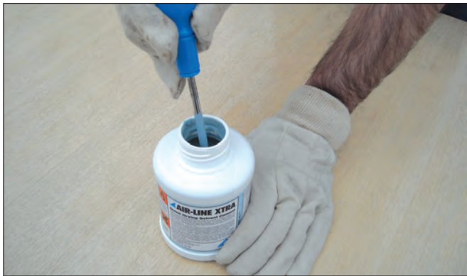
8. Stir solvent cement.
