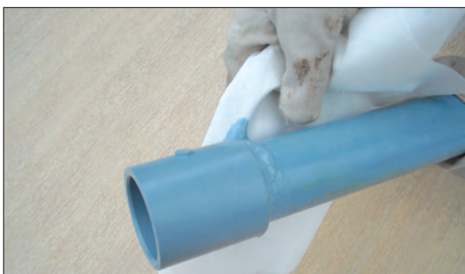
11. Cement will form a neat-bead. Wipe off excess cement with a lint-free cloth.
