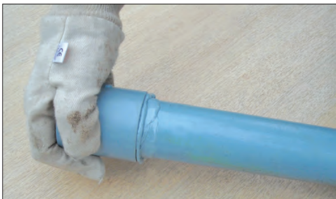
10. Push fitting home and hold for a few seconds.
