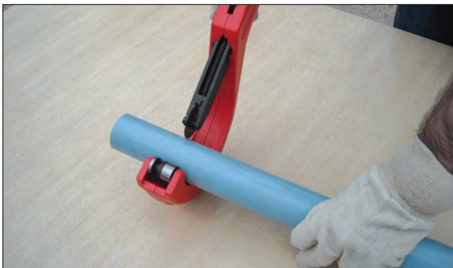
2. Cut pipe to required length.
