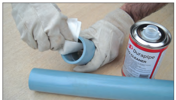
7. Clean pipe and fitting with eco cleaner.
