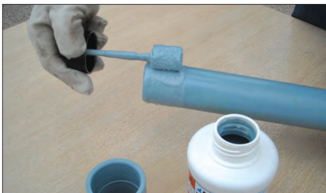
9. Apply cement to pipe and fitting.
